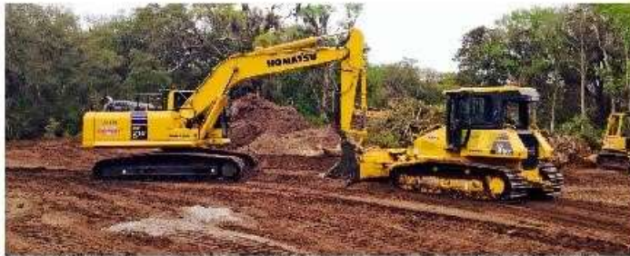
A construction project involving soil disturbance
