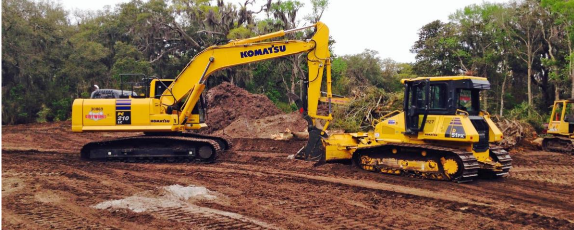
A construction project involving soil disturbance
