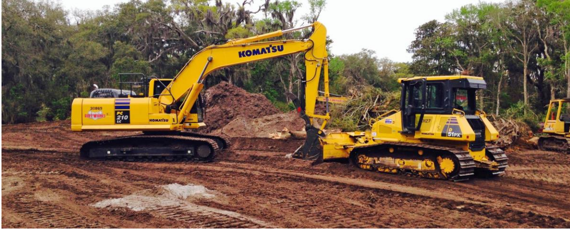
A construction project involving soil disturbance
