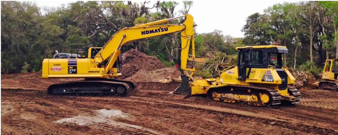
A construction project involving soil disturbance
